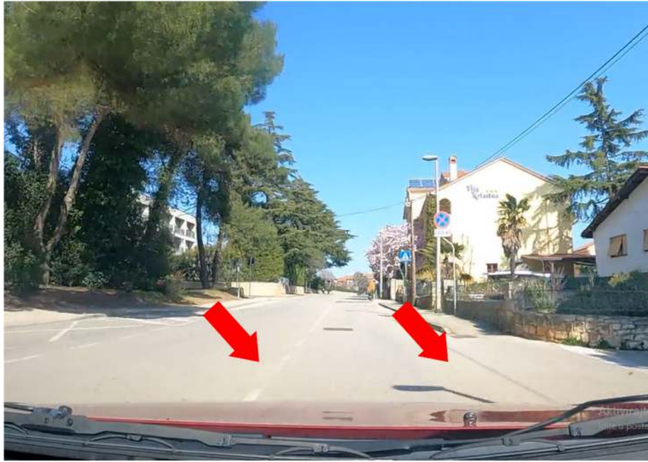
Figure 36 - Faded center line and missing edge line
