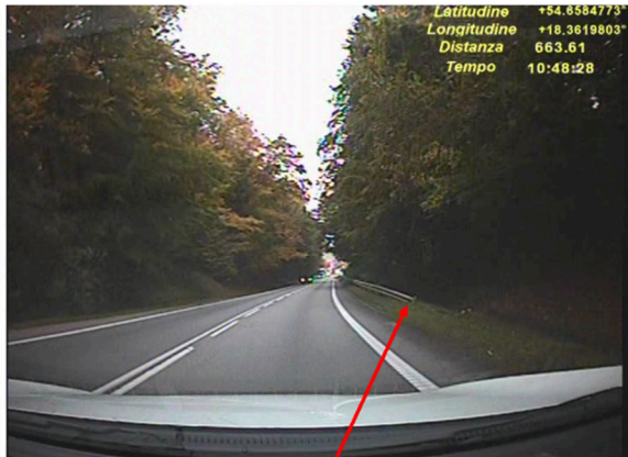
Roadside barrier with no breakway terminal
